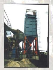
**Project:** Dedusting system on a Asphalt mixing plant - Varna,BG
